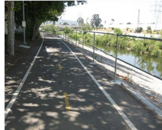
Reach 3 at Marsh Street Park
