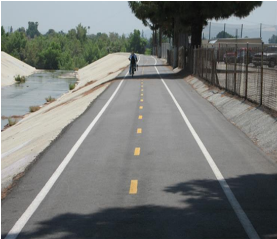
(a) Looking downstream toward confluence – trapezoidal channel with no separating fence
