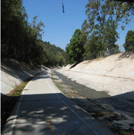
(a) Bike path along channel bottom at Hermon Park
