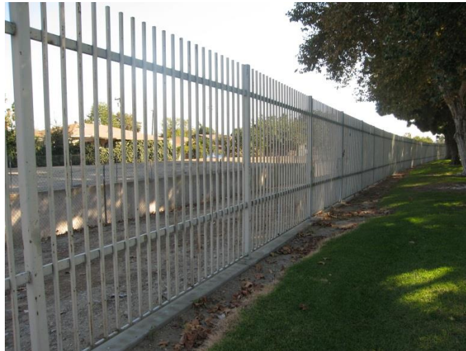
FIGURE 5-3.13: SAWPIT WASH SEPARATED FROM PAMELA COUNTY PARK BY TWO LEVELS OF FENCING
