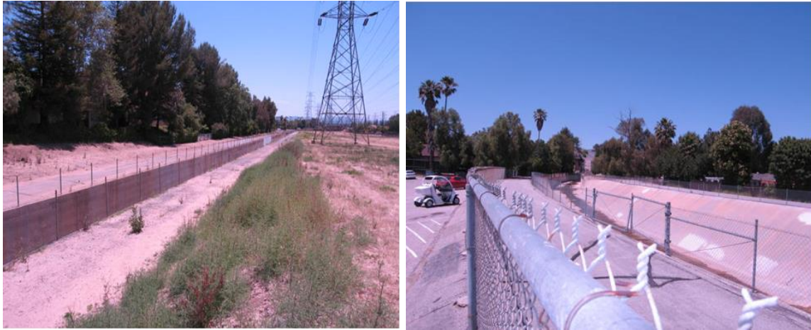
(a) At Northridge Recreational Center
