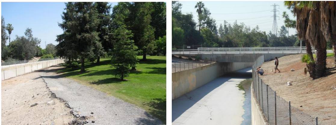
(a) Eaton Wash at the boundary of Gwinn Park
