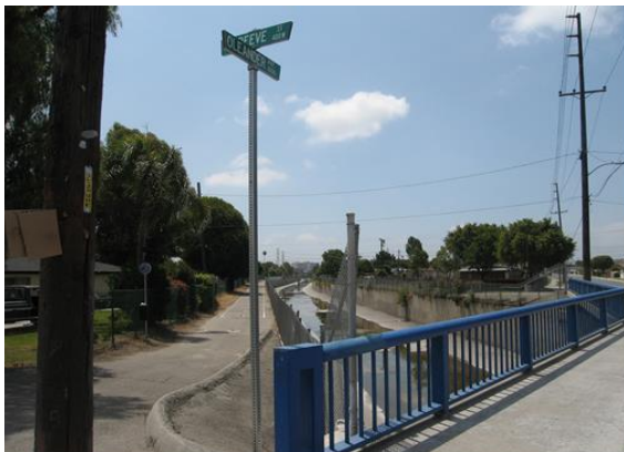
(a) Upper segment at Reeve St/ Oleander Ave.
